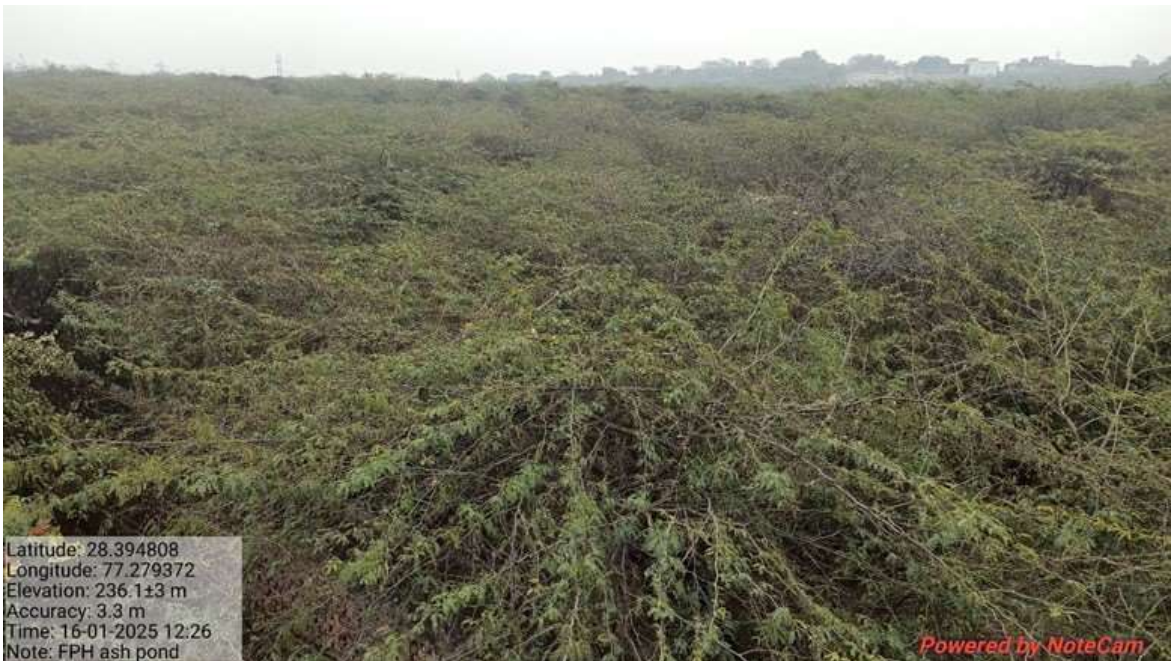
Photograph of Old Ash Dyke of FTPS
