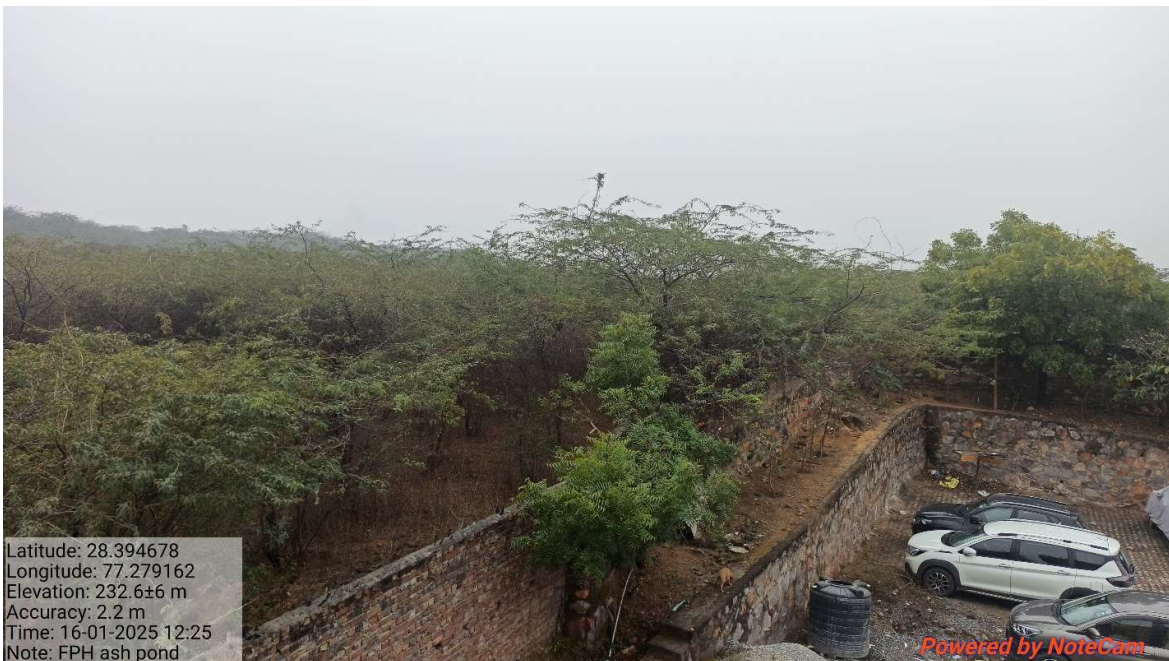
Photograph of Old Ash Dyke of FTPS
