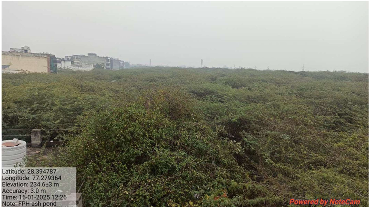
Photograph of Old Ash Dyke of FTPS
