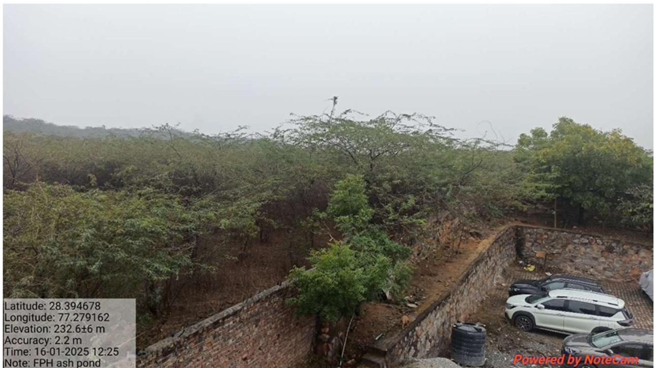
Photograph of Old Ash Dyke of FTPS
