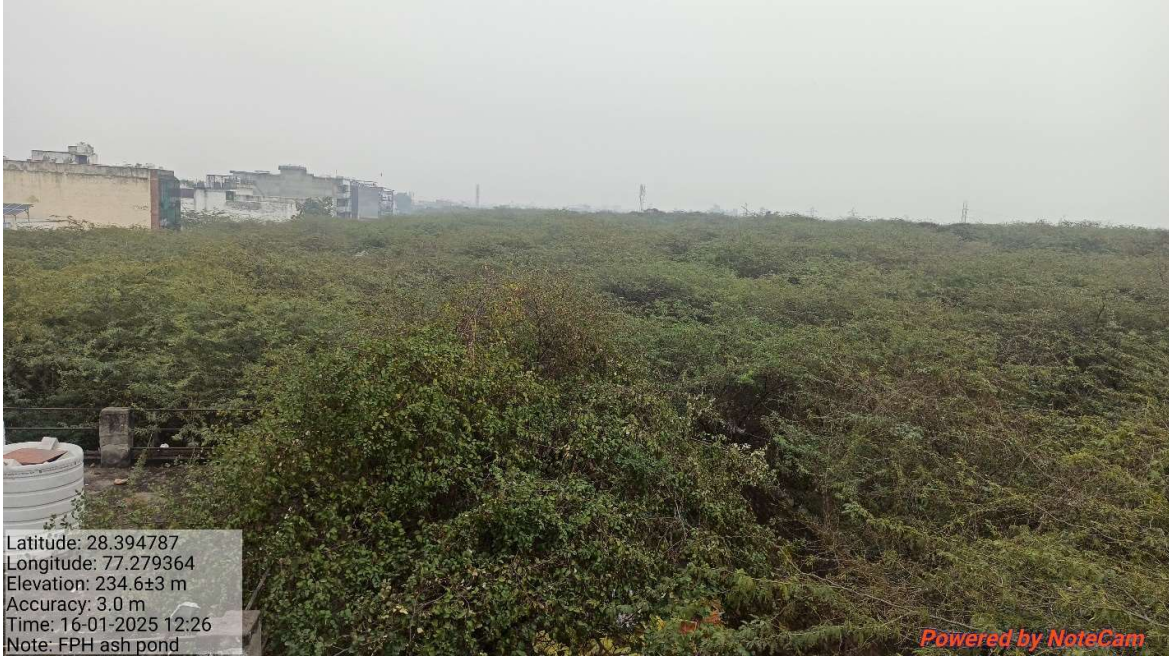
Photograph of Old Ash Dyke of FTPS
